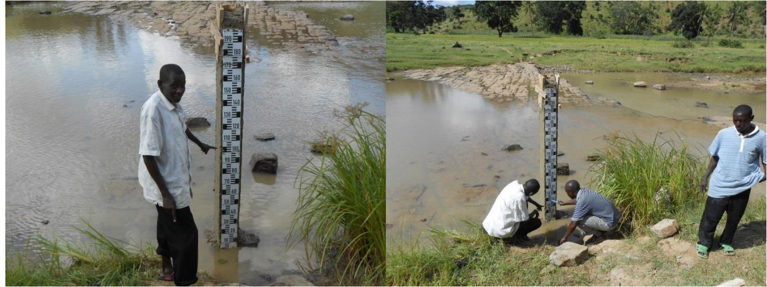
b) Concrete post installed at Mwache 3 MB02 Gauge reader being trained on reading RGS in Athi Catchment
